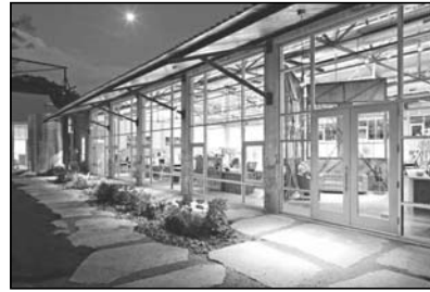
Photo by Chris Cooper Large concrete flagstones in the SoFlo Studios courtyard are actually remnants of the old warehouse parking lot and driveways.
