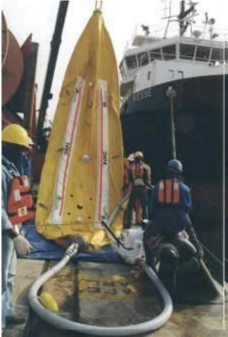
NRC oil spill response team in action
